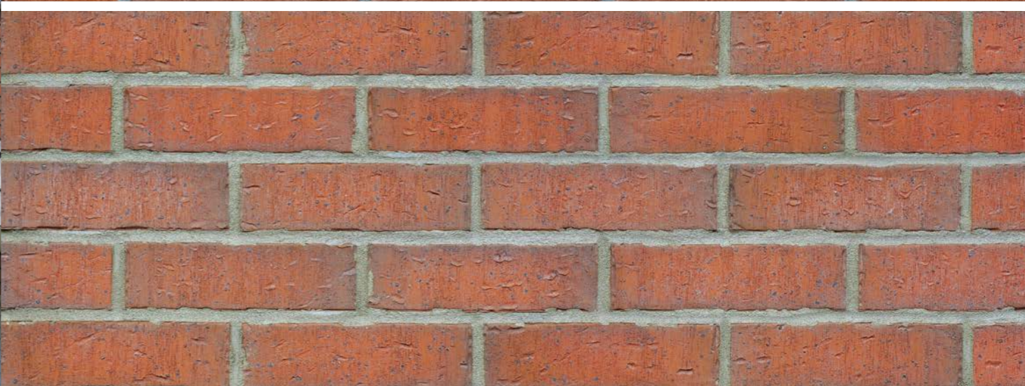
Brick tower HF03
